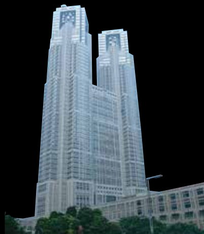
TOKYO METROPOLITAN GOVERNMENT NO.1 BUILDING
